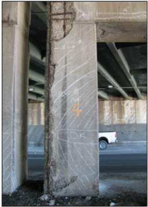
PIER 1 COLUMN 4 NORTH FACE
