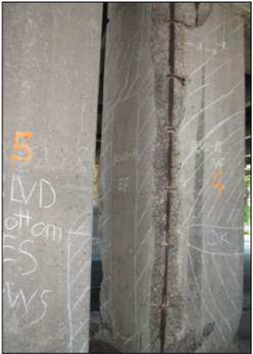
PIER 1 COLUMN 4 EAST FACE
