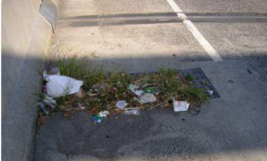
Cleaning Drainage System
