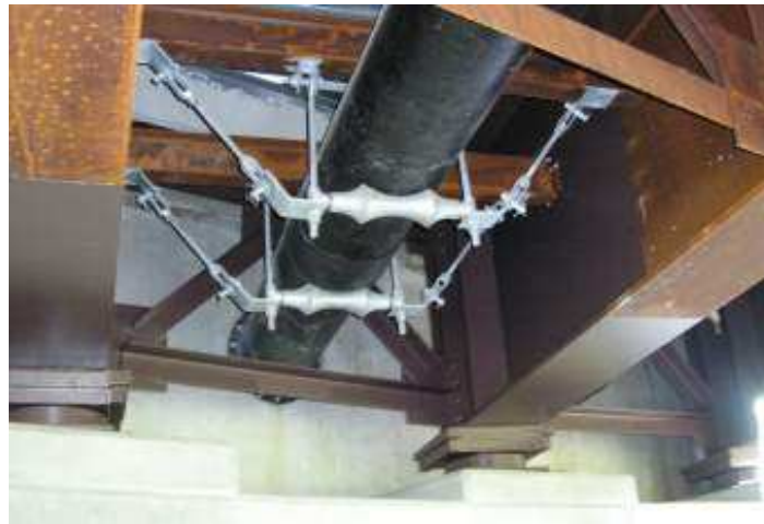
Painting Girder Ends
