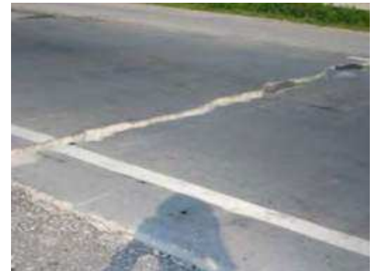
Condition 1. The difference in the height between the roadway and the bridge deck is greater than 1-inch, which might give rise to a hazardous condition leading to potential vehicle damage
