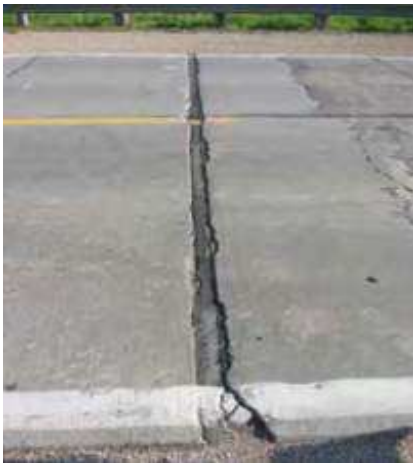
Condition 3. Moderate deficiencies exist, but do not affect the integrity of the structure. The difference in the height between the roadway and the bridge deck is approximately \frac{1}{2} -inch
