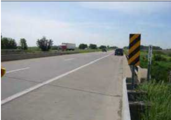
Condition 5. No deterioration other than superficial cracks. The difference in the height between the roadway and the bridge deck is negligible
