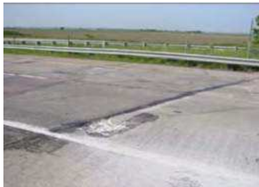
Condition 2. Significant deficiencies exist. The difference in the height between the roadway and the bridge deck is approximately \frac{3}{4} -inch, causing the travelers to experience a significant bump
