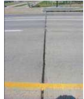
Condition 4. Minor deficiencies may be present. The difference in the height between the roadway and the bridge deck is approximately \frac{1}{4} -inch, causing the travelers to experience a slight bump
